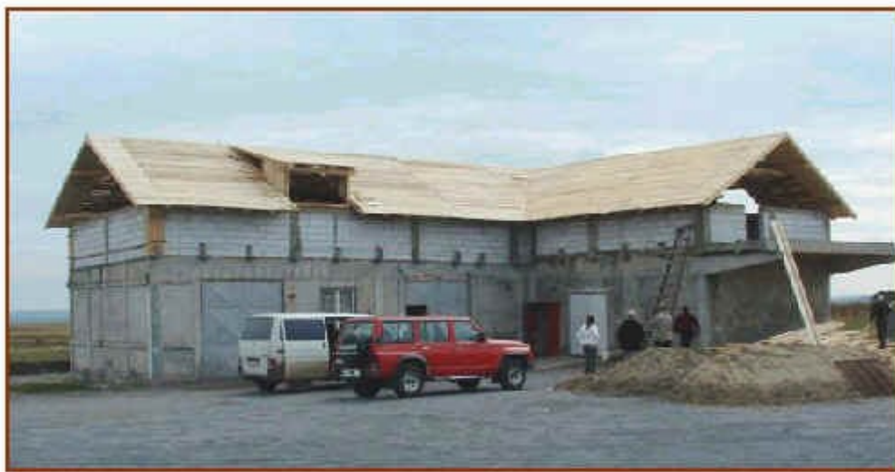
The roof structure nears completion in October 2004
